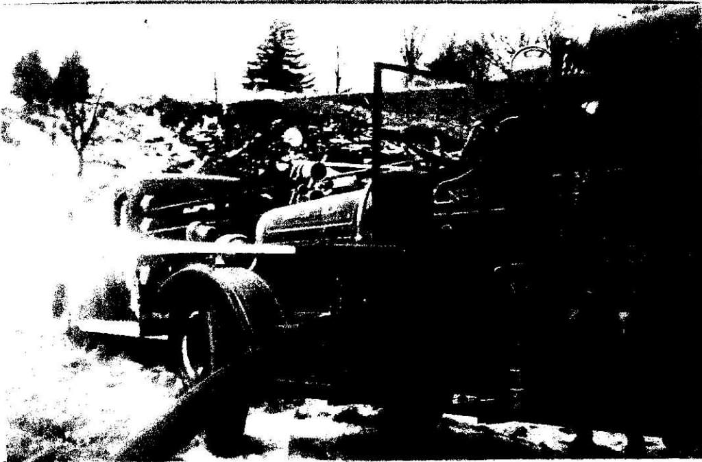
Pumping practice around 1943. The scene is at Hoffa's creek near where the Senior citizens gazebo now stands. The new Ford American LaFrance is just ahead in the picture. Note the homemade windshield, soda acid extinguisher, kerosene lanterns, and tiny 6-volt siren on the fender. The fancy hand holds on the side of the driver's seat and the curved handhold in front of the windshield were used by firemen while standing on the running board. The truck was bright red and the gold leaf lettering and decorating was extensive.
