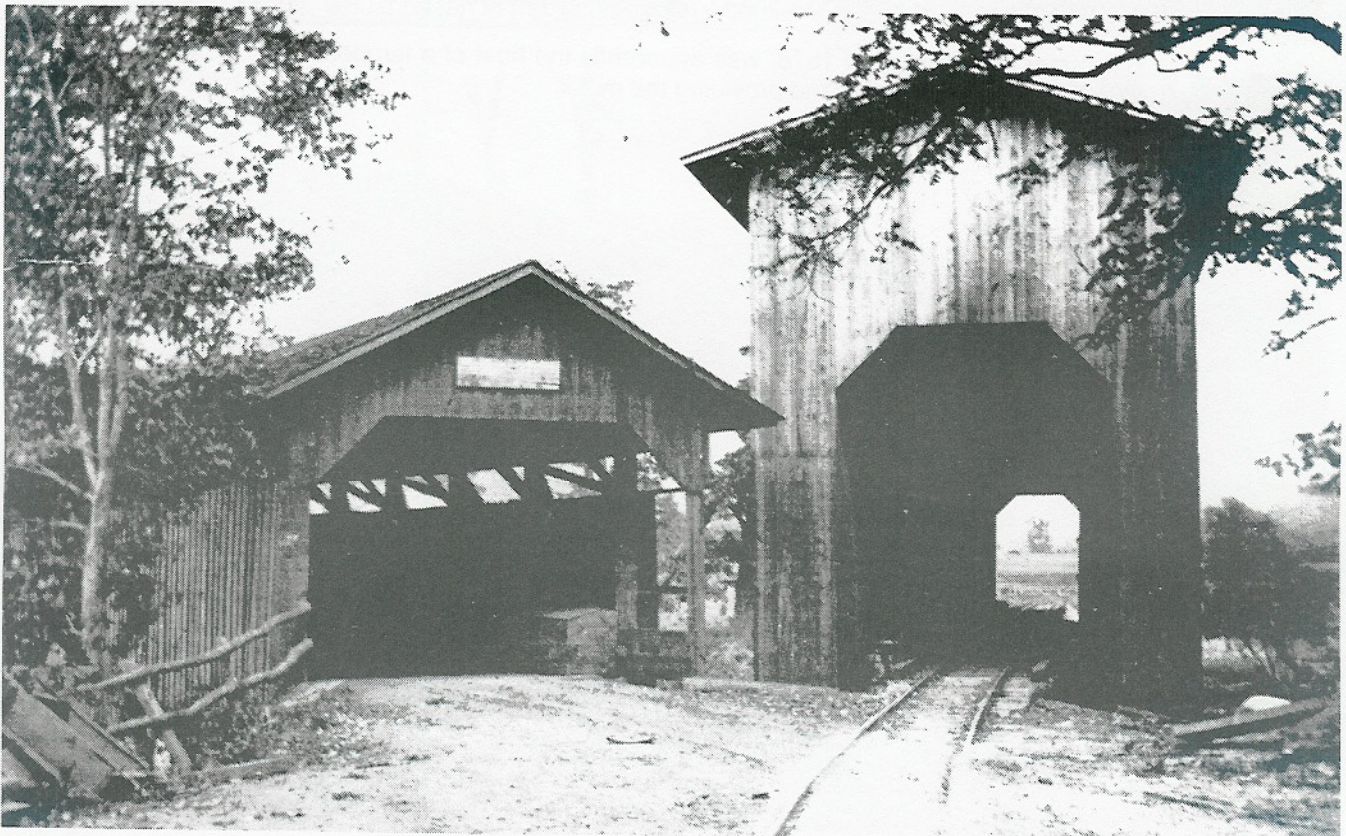
Side by side, an unusual arrangement of covered bridges cross the Loyalsock below Hillsgrove. The traffic bridge, left, was in service until the 1920's (exact date unknown), while the wooden railroad bridge collapsed and was replaced by an iron truss bridge, illustrated elsewhere in this book.
